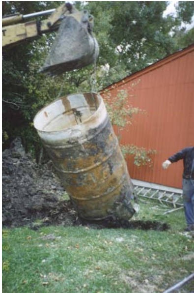
Removal of well pit cribbing
