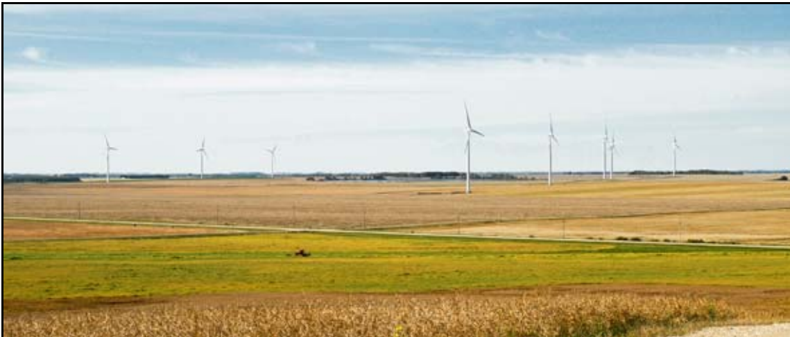
Image 11 - Panoramic view – St. Leon Wind Farm
