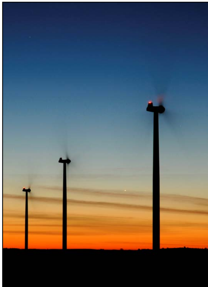
Image 7 – Wind Turbine Safety Lighting
