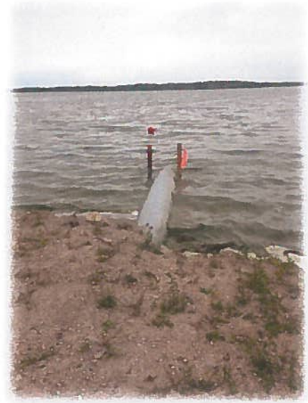
Figure 4: Existing Provisional Outlet
