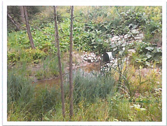
Figure 7: Culvert East Side of Keeseekoowenin Reserve (Crossing #9)
