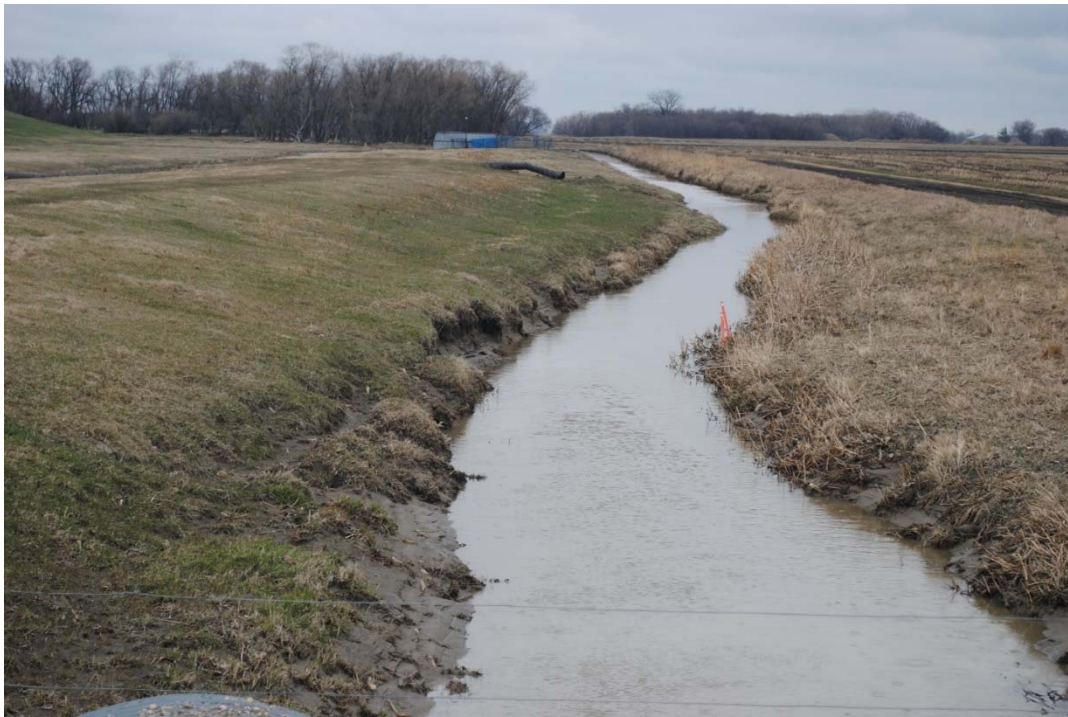
Figure 16 - Shannon Creek - NE 3-4-5 W - Looking East - Channelized and Dyked
