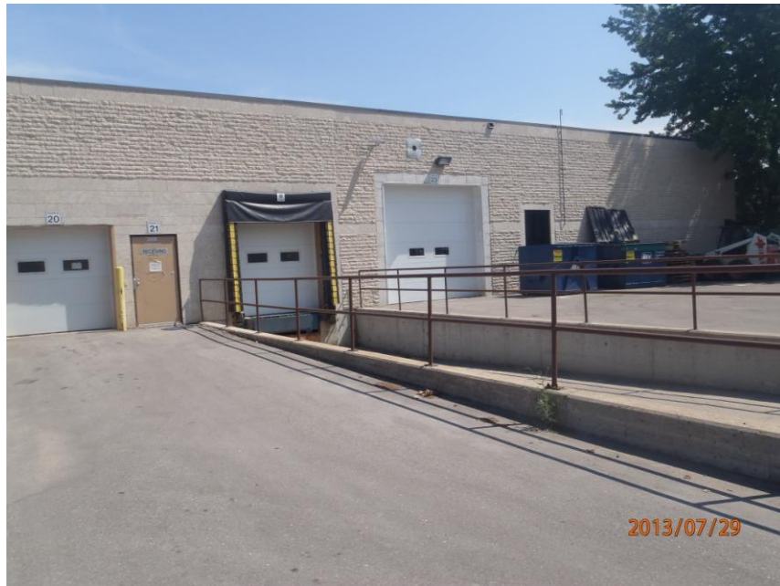
PHOTOGRAPH 2: Looking east, west wall of Site building, loading and unloading zone.
