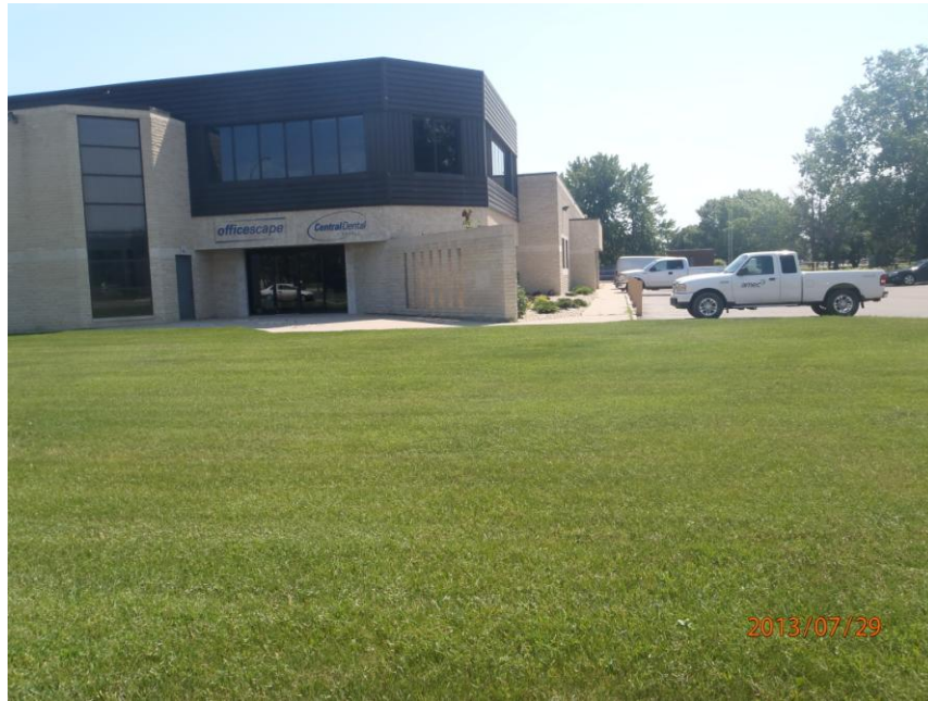
PHOTOGRAPH 1: Looking south, exterior of building.
