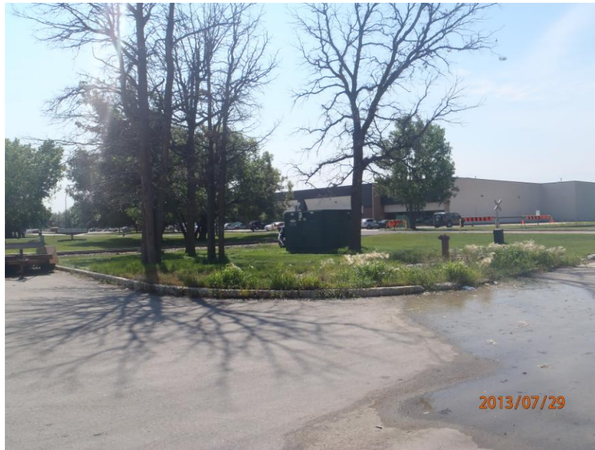
PHOTOGRAPH 5: Facing southwest from southwest corner of Site building, showing surrounding land.
