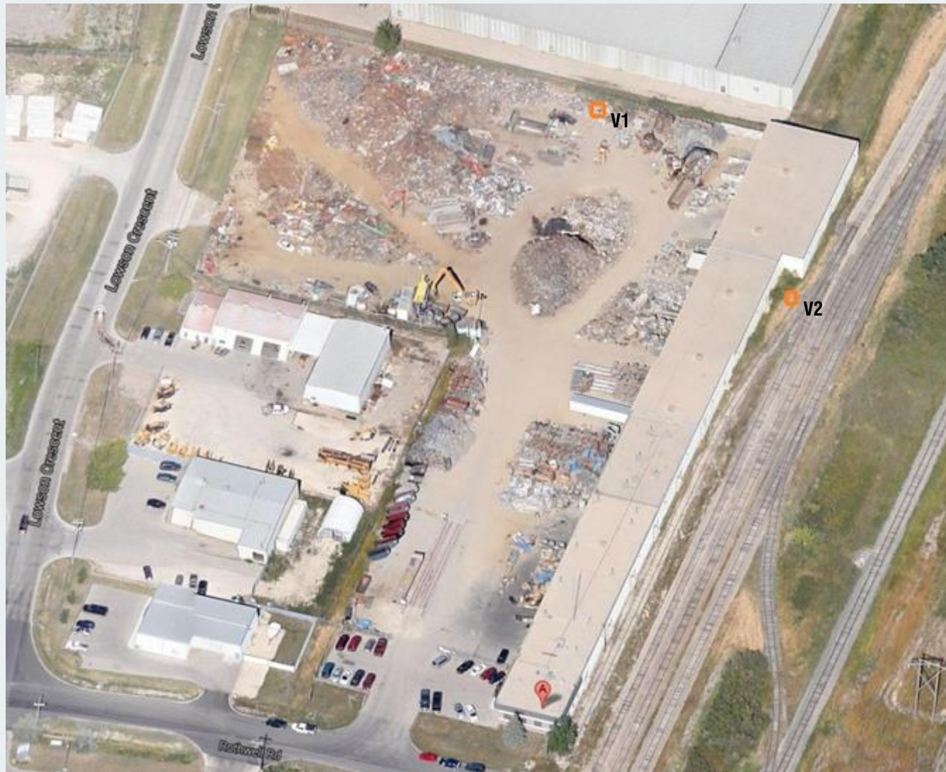
FIGURE 3: ON-SITE VIBRATION MEASUREMENT LOCATIONS
