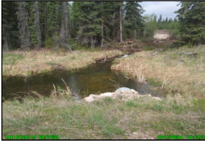
Photo 1: Stream crossing HWYAN, looking west.
