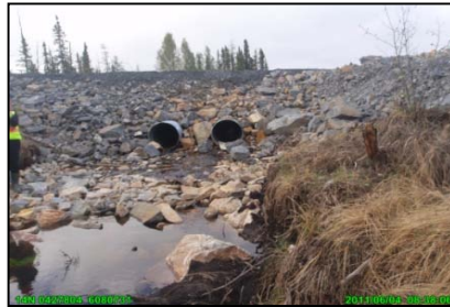
Photo 3: Stream crossing LR01, looking south
