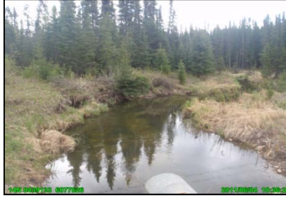
Photo 2: Stream crossing HWYAN, looking east (downstream).
