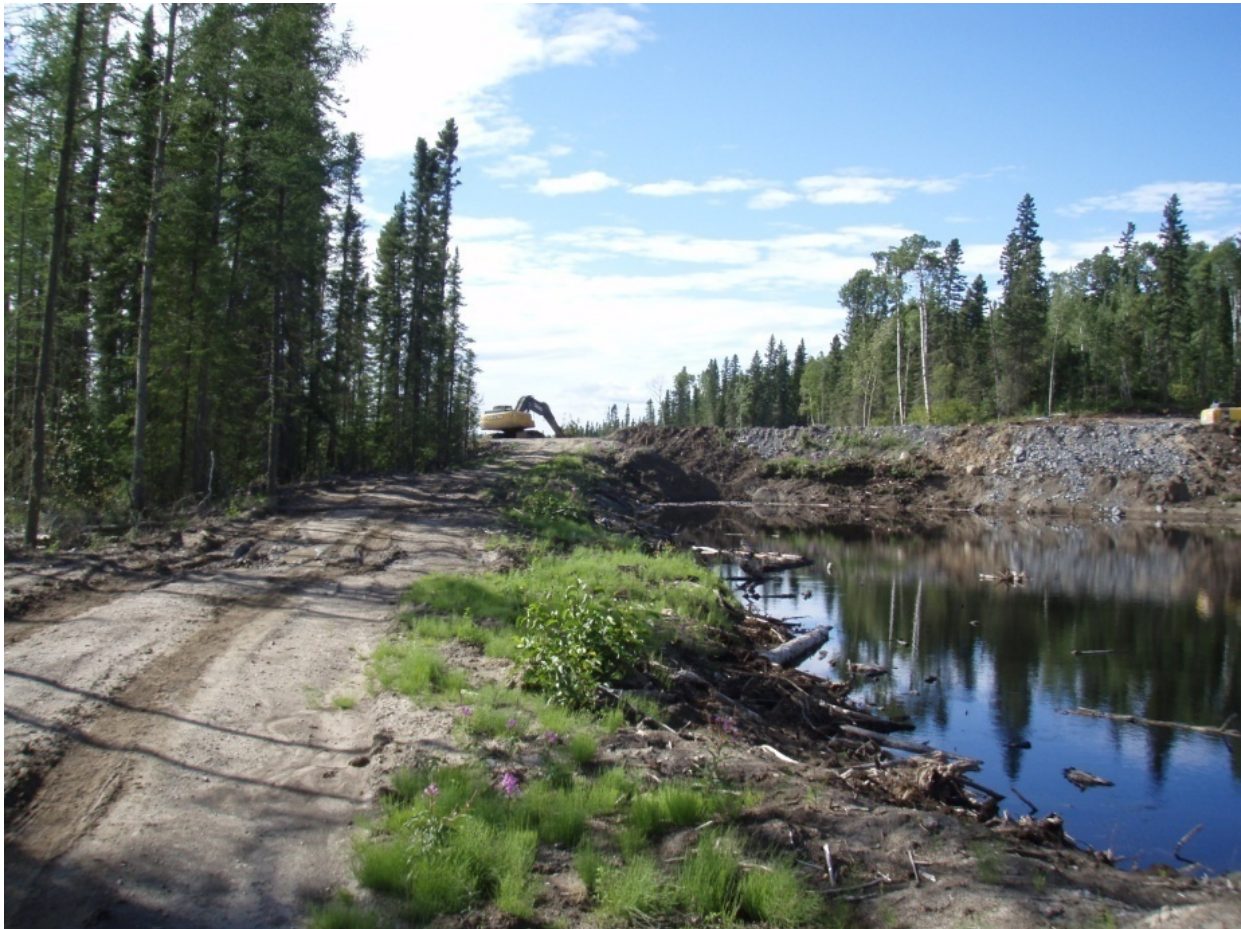
Figure 27: Cleared Roadway Adjacent to the Drainage Channel
