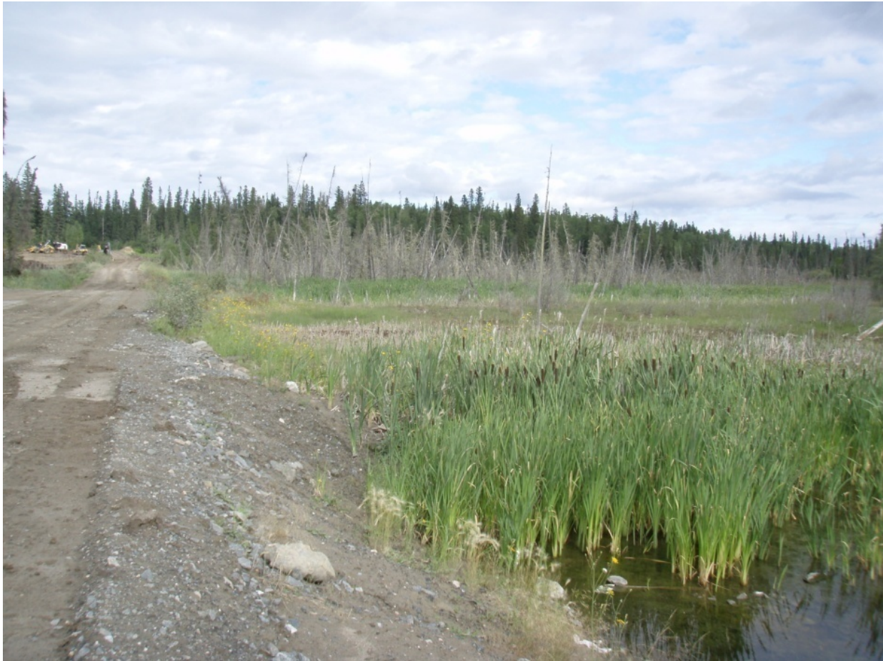
Figure 26: Road Adjacent to Drainage Channel
