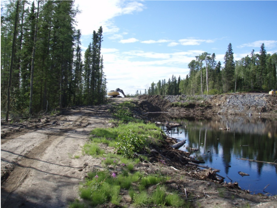
Figure F8: Road north of Drainage Channel, Proposed Pipeline Route
