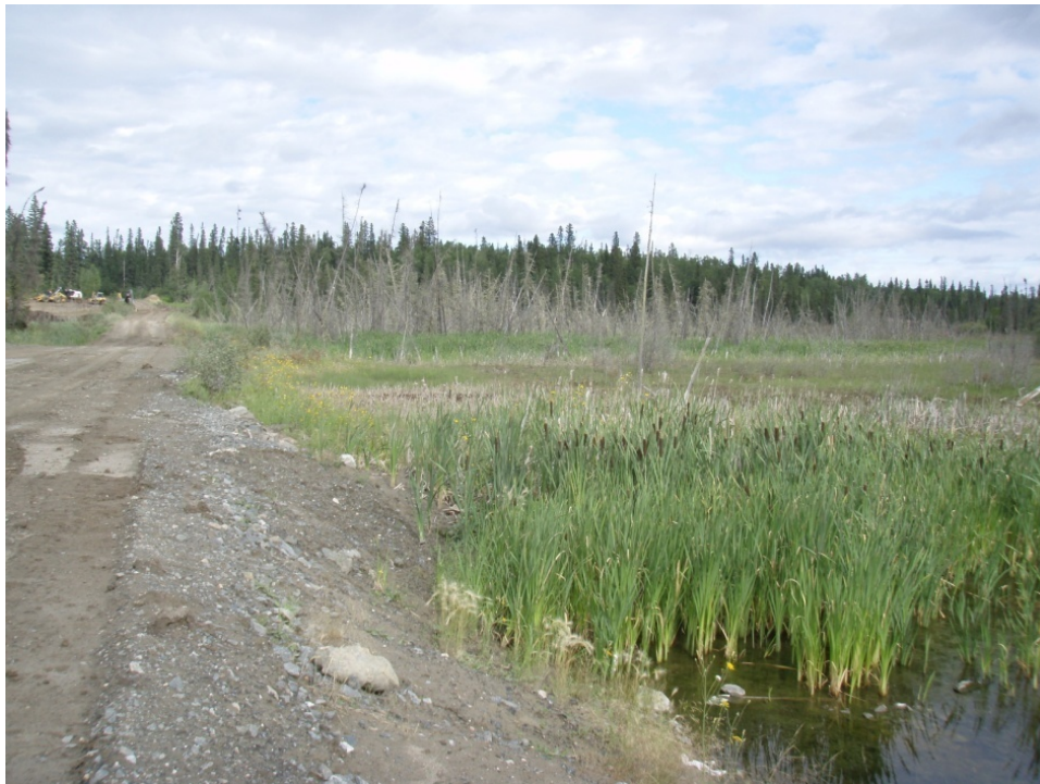
Figure F6: Road Adjacent to Drainage Channel
