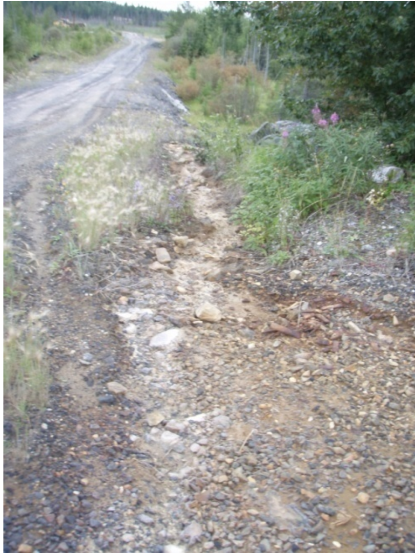
Figure 15: Surface Runoff from the Northeast Side of the Arsenopyrite Residue Stockpile
