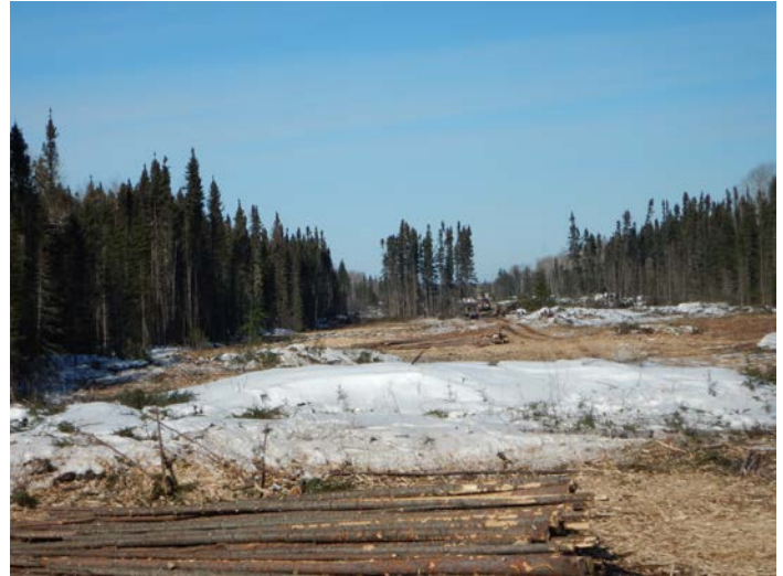
Photo 1: Right-of way during the vegetation clearing process
