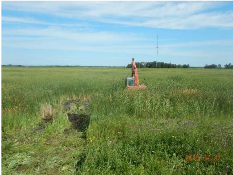
Photo 1. Excavator sampling Oakbank lagoon cells.
