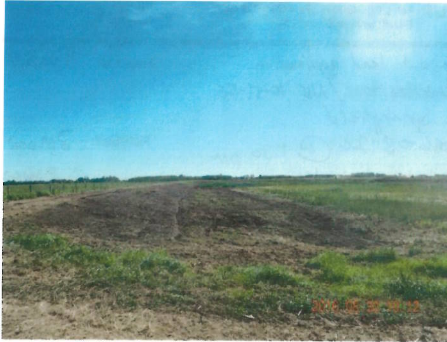
Photo 5. Completed North Cell at Dugald lagoon
