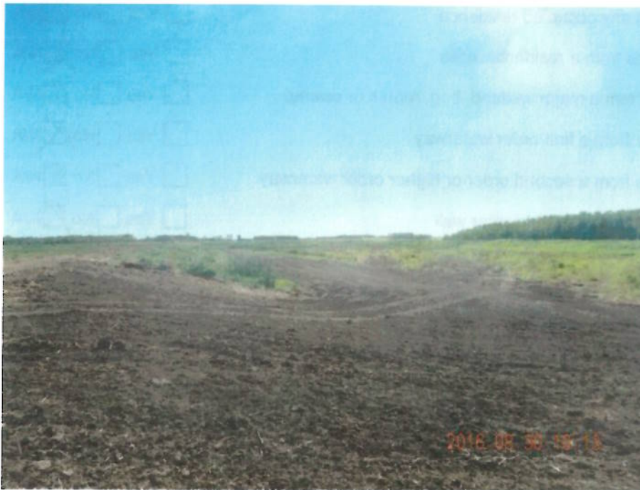
Photo 6. Completed South Cell at Dugald lagoon
