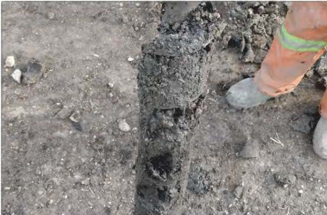
Photo 2: Clay (Fill) Stockpiled Above Original Ground at Borehole 22BH01
