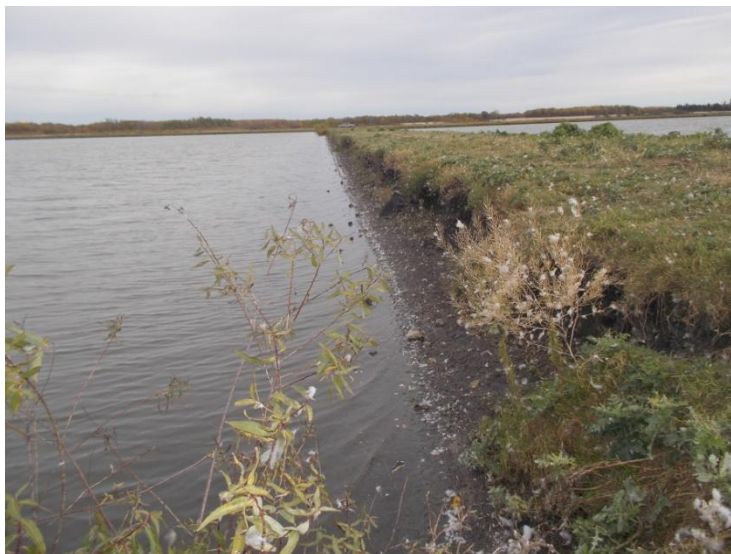
Figure 1 – Storage Cell 2 dike at the Storage Cell 1 – 2 intercell dike
