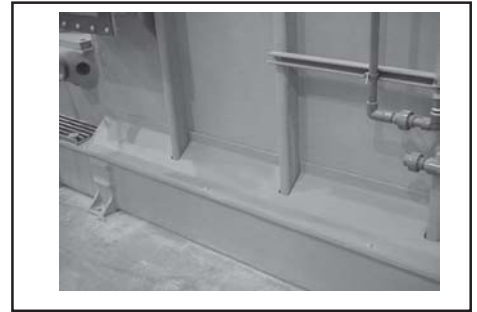
Secondary Containment-Rain Covers
