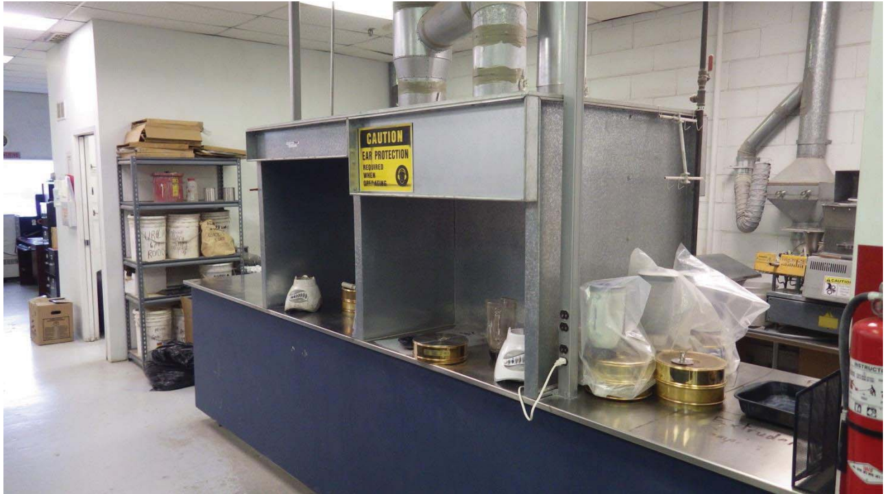
Photo 9. Fume hood in powder coatings lab.
