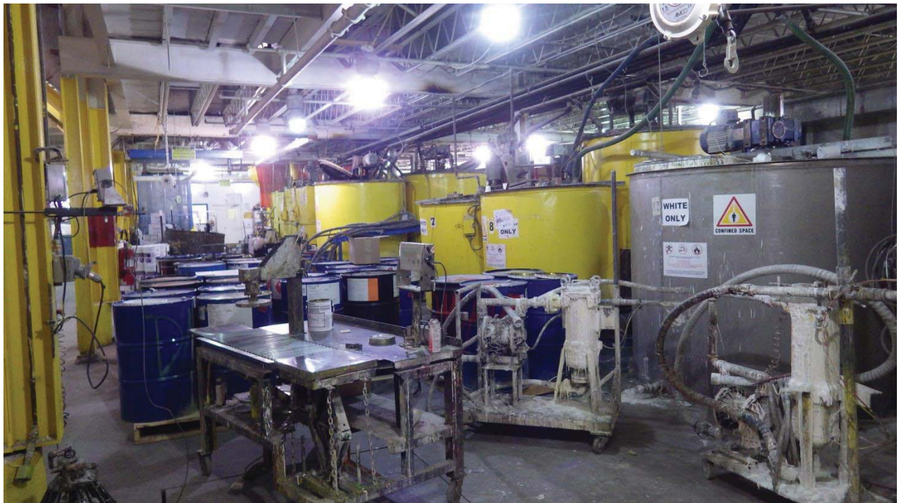
Photo 16: Liquid paint production area beneath the mezzanine.
