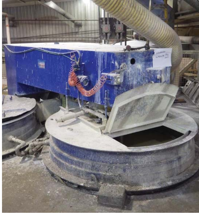
Photo 15: In-floor liquid paint coatings process tank (mixer) on the mezzanine.
