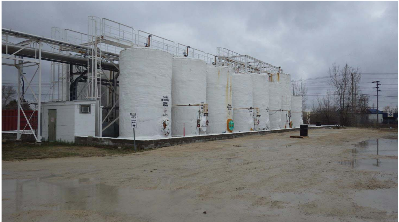
Photo 7. North view of spill contained tank farm.
