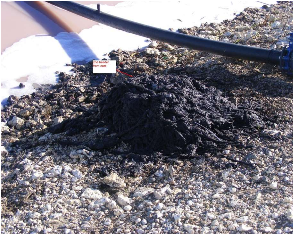
Figure 3.14: Debris Accumulation in Cell 1
