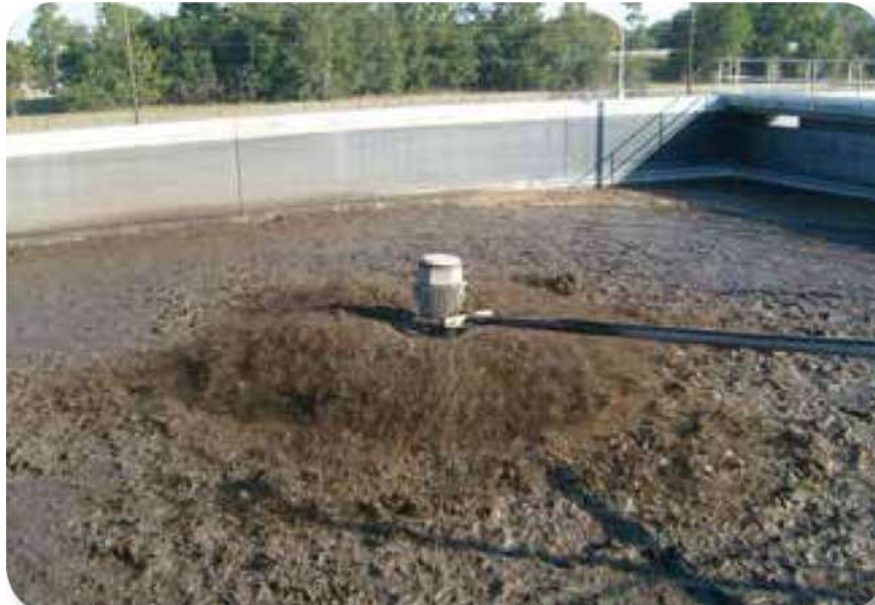
Figure 3.11: Floating Mechanical Mixer/Aerator (Image from Aqua-Jet)
