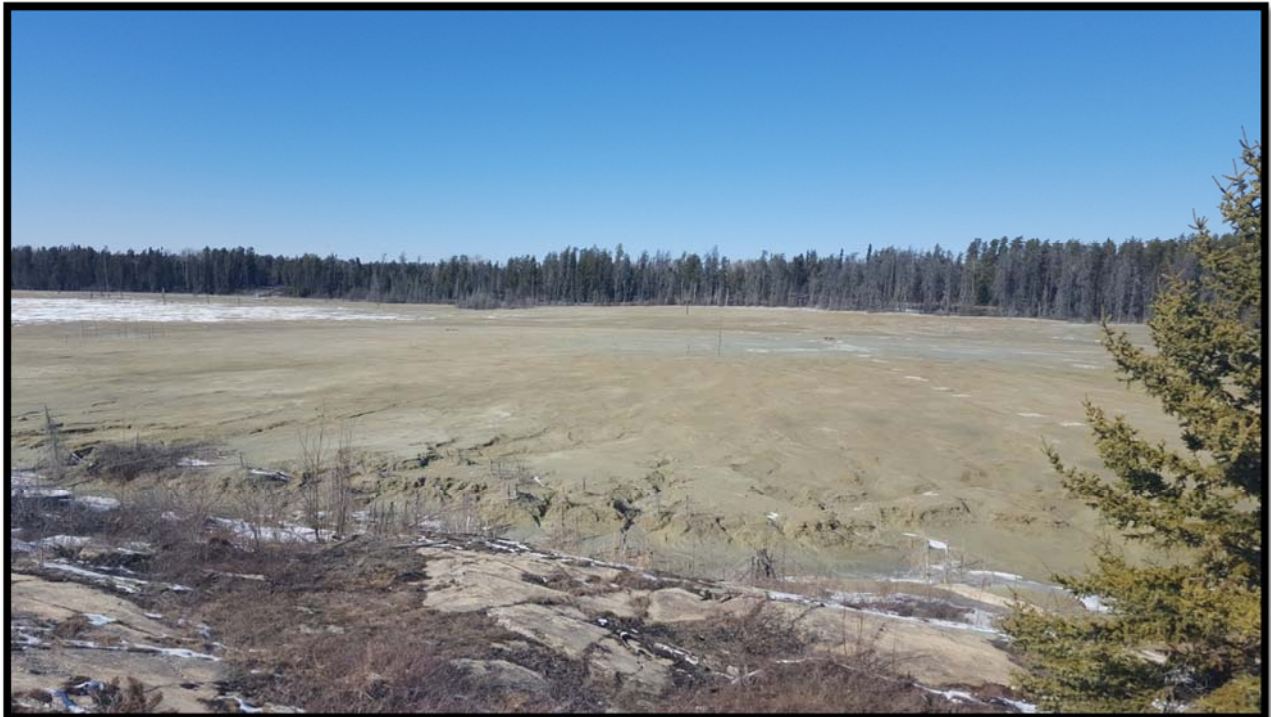
Figure 2: Recent Photograph of the Existing Tailings Pond Taken April 2016
