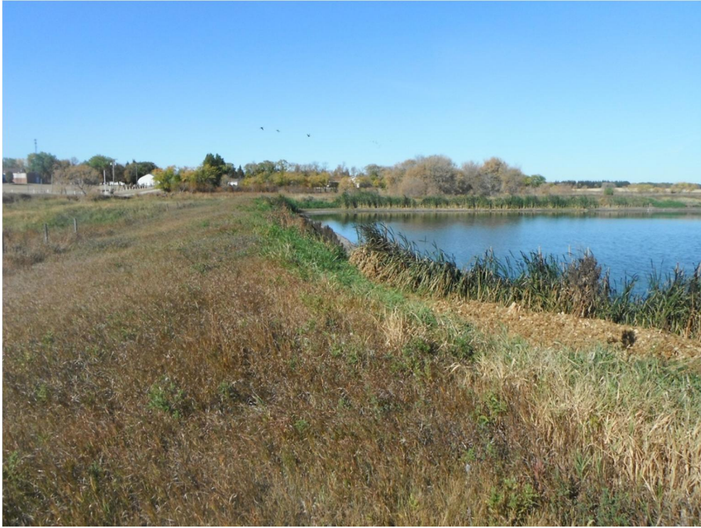
Perimeter Fencing seen on left; Lift Station in the background
