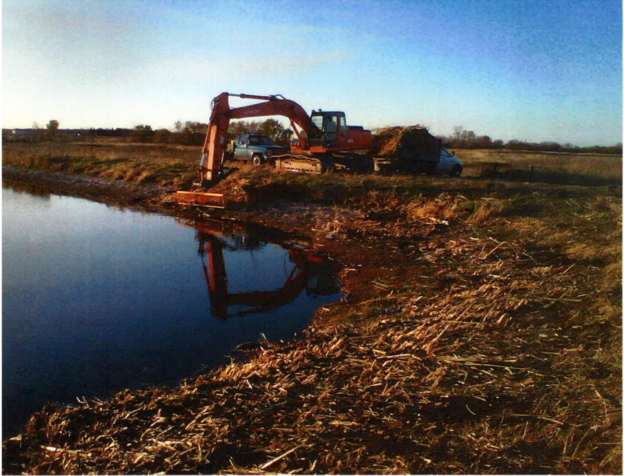
Clearing of excess growth at Baldur lagoon (2011)
