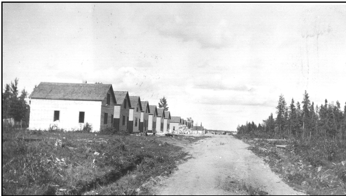
Company houses of The Pas Lumber Company, on First Street, The Pas, c. 1912. Source: P.A.M.
