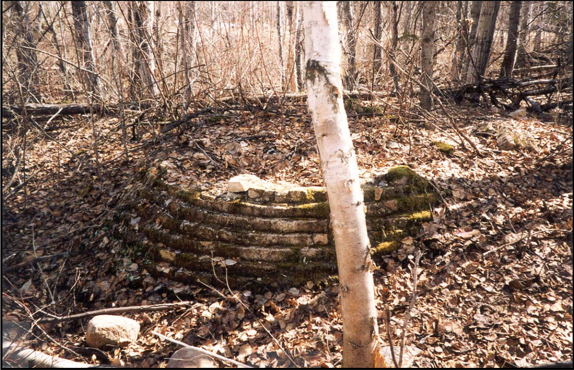
Remnants of refuse stack used to burn the bark and trimmings at the Red Deer Lake mill, 1998. The fire transformed water into steam to power the sawmill. Source: HRB.
