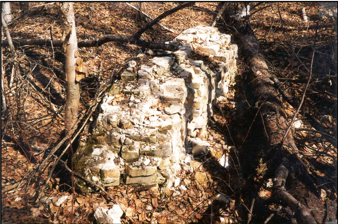
Remnants of refuse stack used to burn the bark and trimmings at the Red Deer Lake mill, 1998. The fire transformed water into steam to power the sawmill. Source: HRB.
