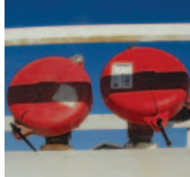
Plastic valve covers and ties offer a quick visual clue to tampering.
